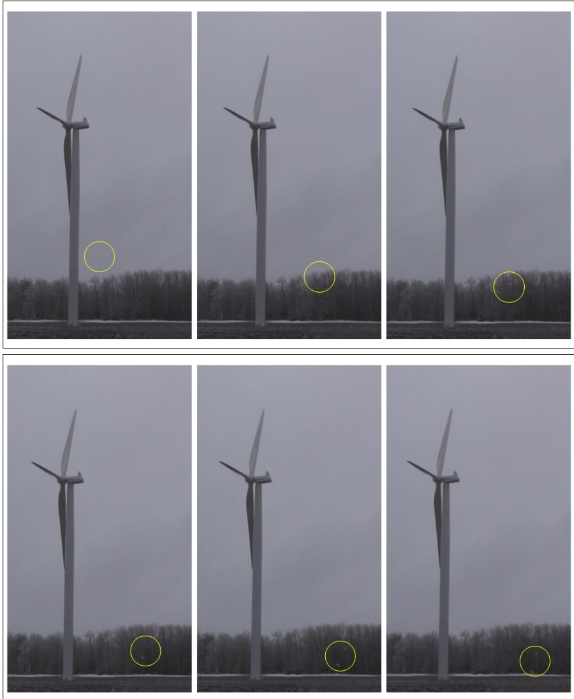
Figure 11. Time Lapse – Circled Ice Falling from Stopped Turbine in Bruce County
